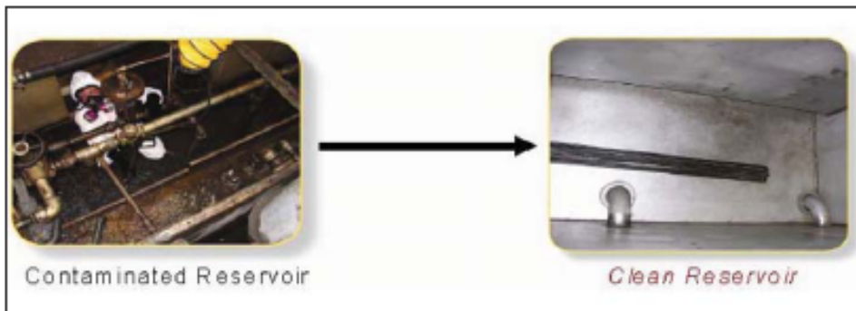
Figure 4: Results of a reservoir decontamination
