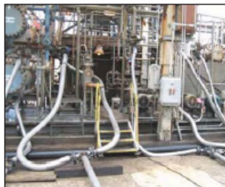
Figure 3: During decontamination of a lube oil system, multiple jumpers and flushing loops are required to isolate every part of the system
